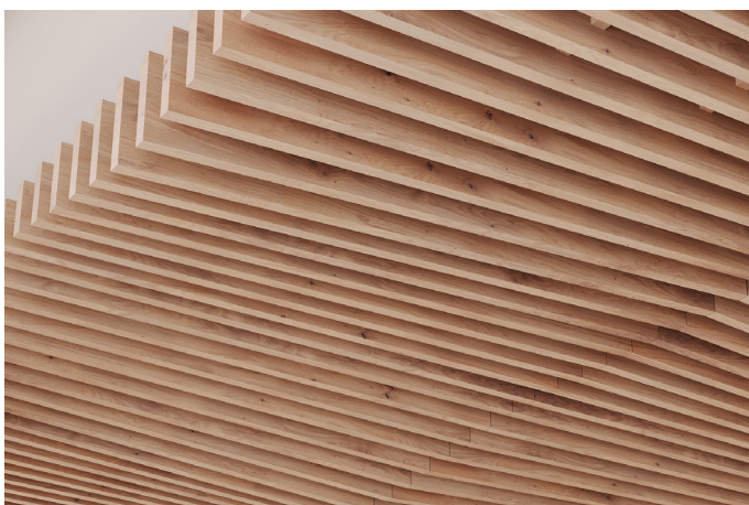
Rail, Lines Ceiling Frames in Fumed Oak
