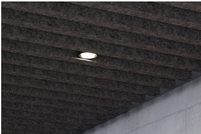
Truss Ceiling Baffles in Thicket
